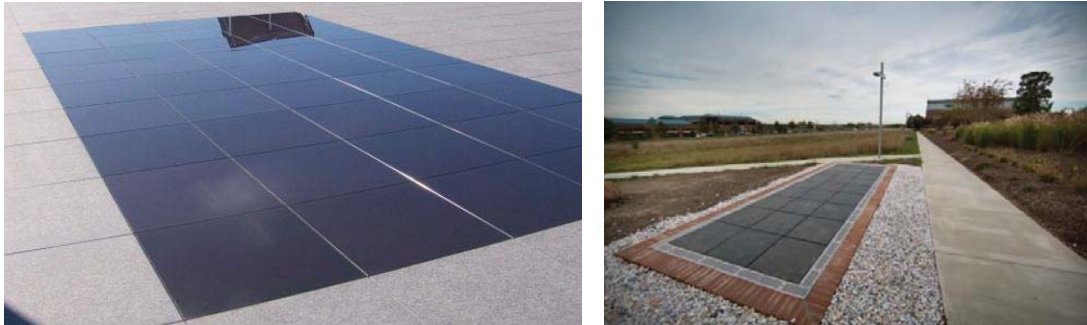
Figure 2 A walkable PV pavement system
